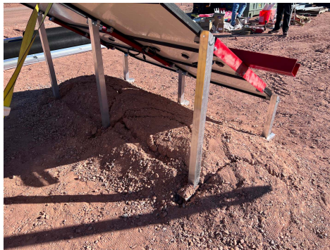
PHOTO 14: Ballast and frame after completion of testing
